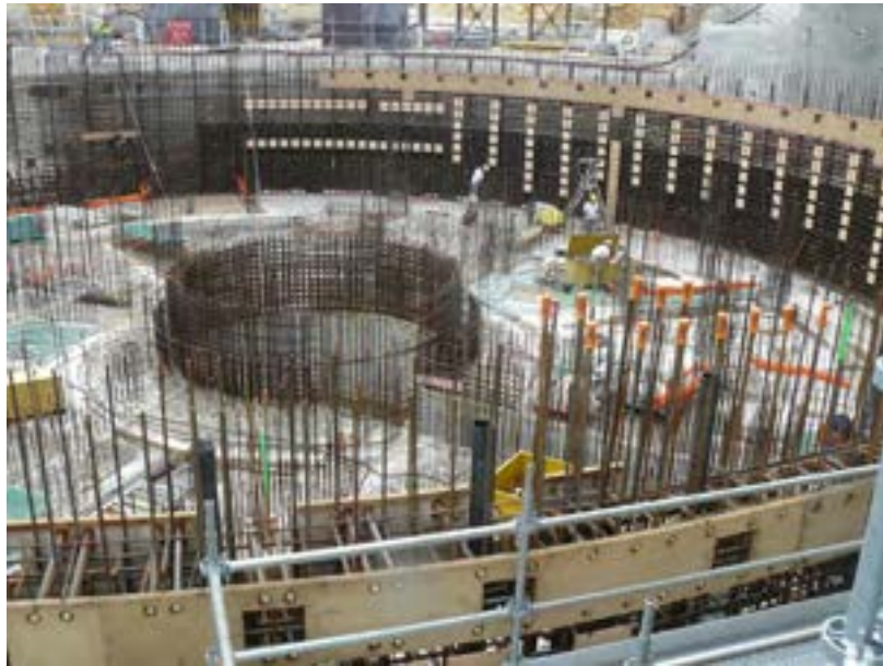
Figure 4: JHR construction site in 2011, reactor building.
