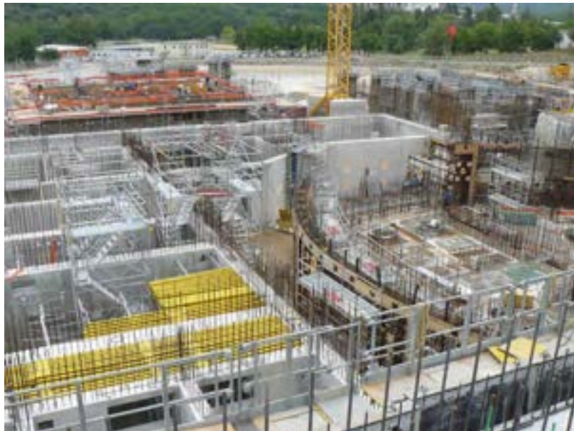
Figure 5: JHR construction site in 2011, nuclear auxiliaries building.
