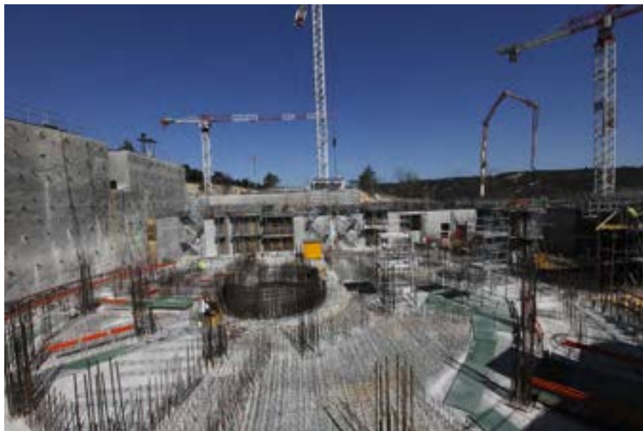
Figure 3: JHR construction site in 2011.
