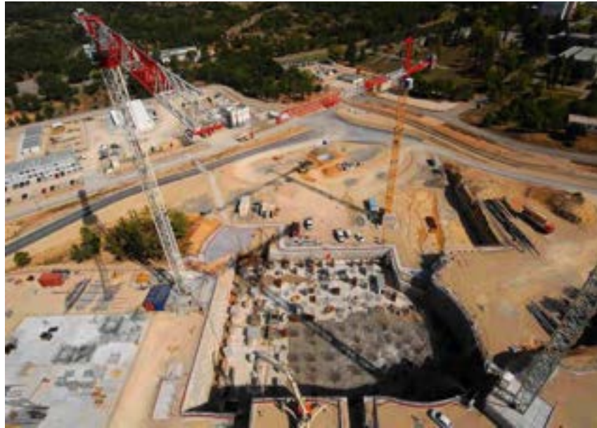
Figure 2: JHR construction site at the end of 2009.
