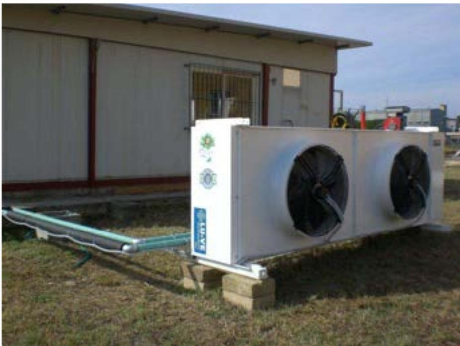
*Fig. 21 – Dry-Cooler modello AERMEC CSE 314 BM*
