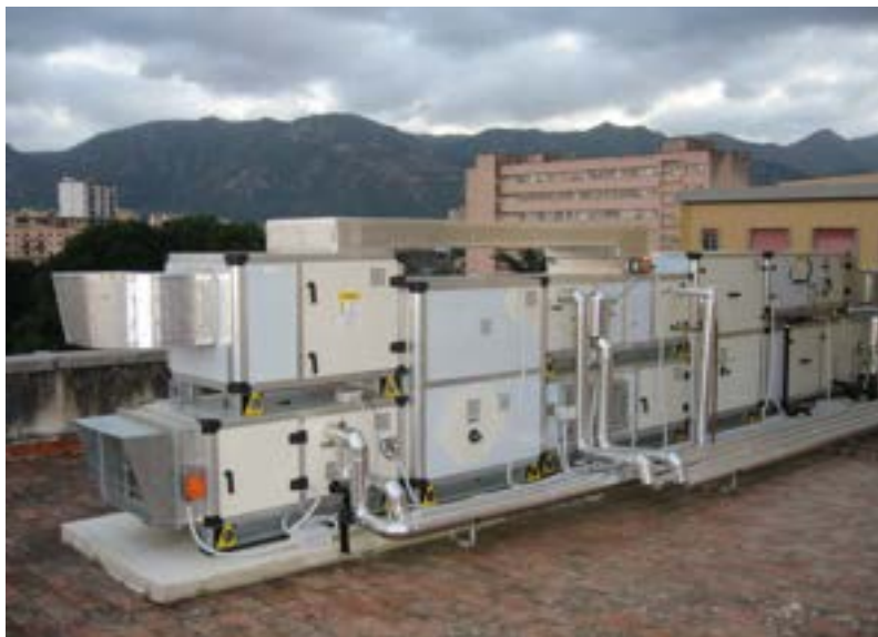
Figure 5.11. Example of a desiccant air-handling unit with integrated heat pump and two additional coils (nominal air-flow 1500 m 3 /h). (source: Dept DREAM, University of Palermo, Italy)
