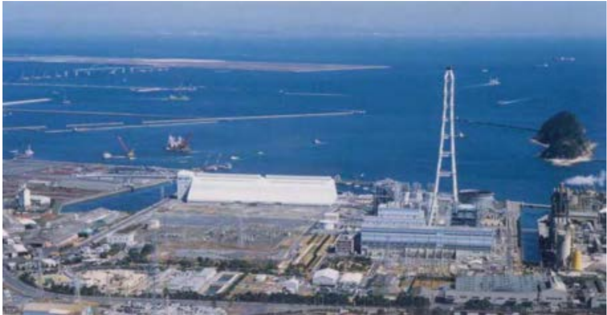
Figura 4.12. Impianto PFBC Karita Therma Power Station 32 .
