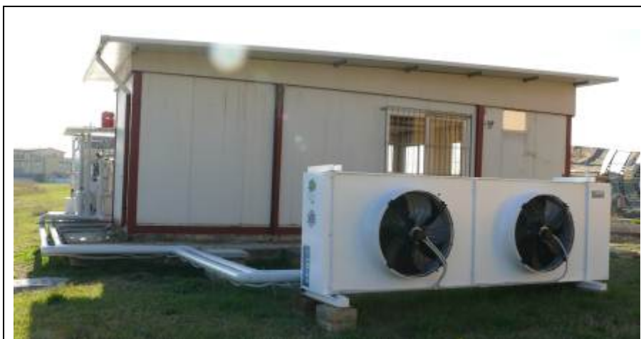
FIGURA 1.37: Dry Cooler SAL8S 2122 C V
