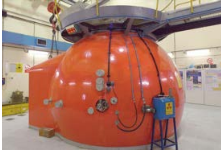
Figure 3.1 - TAPIRO reactor room.
