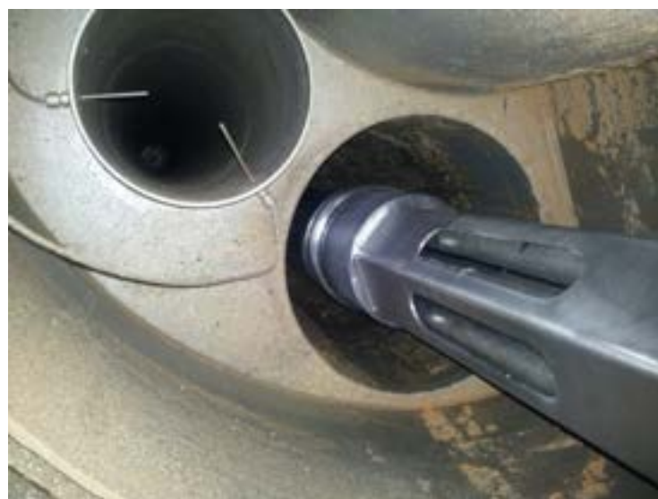
Fig. 16 – TCs arrangement at the outlet section of the riser
