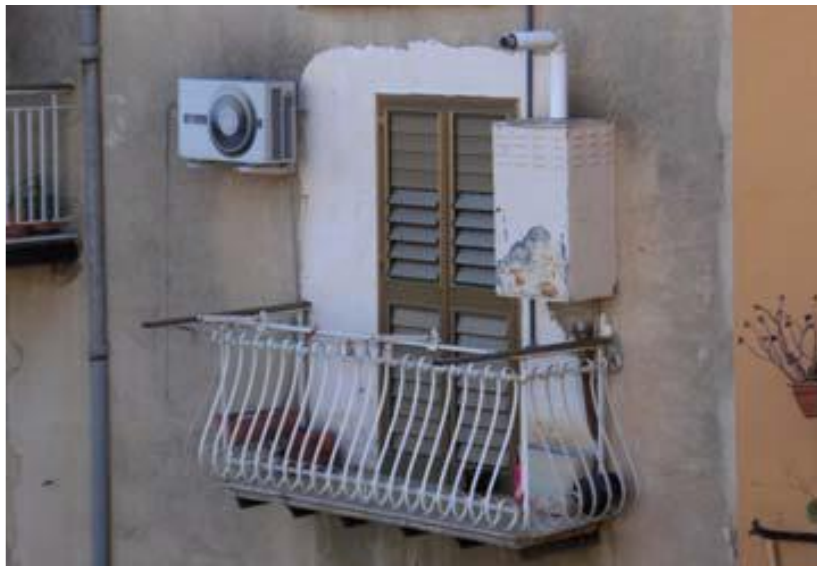
Figure 2: Typical individual heating and cooling systems in the southern Italy (Sven Werner) [10].
