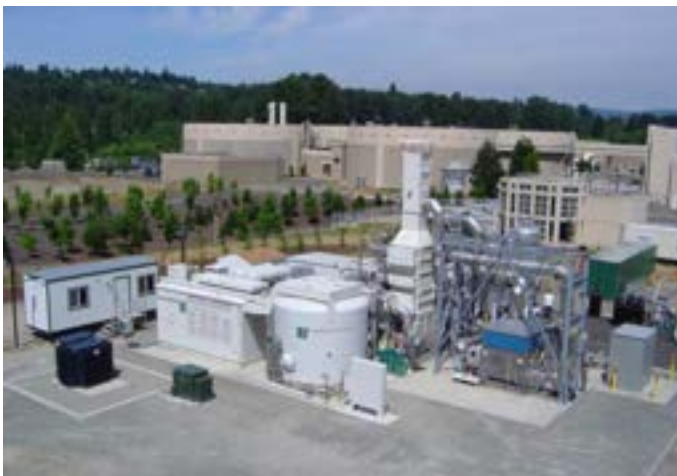
Figure 2. King County Power Plant (courtesy of FCE)
