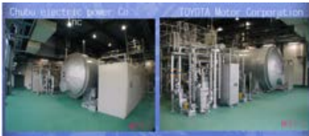
Figure 16. MCFC operated on alternative fuels, at the 2005 Aichi Expo, Japan (courtesy of CRIEPI)
