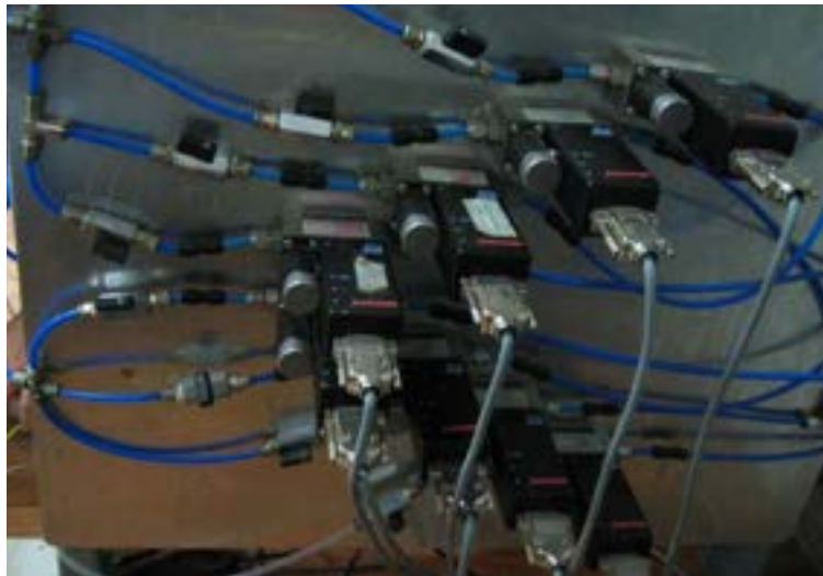
Figura 6. Flow Meter Controllers.
