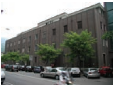
View of the building before retrofit
