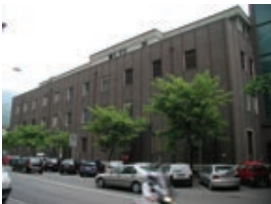
Fig.5: View of the building before retrofit
