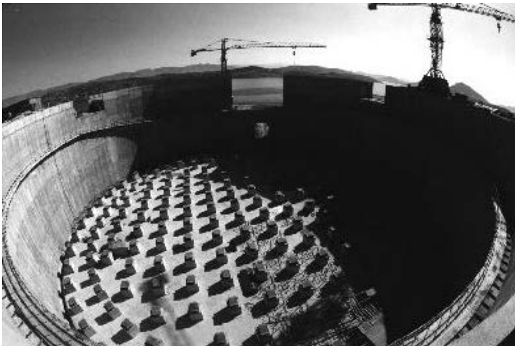
Fig.1 - LNG Tank in Revithoussa island in Greece during construction (Constantinou 1997)
