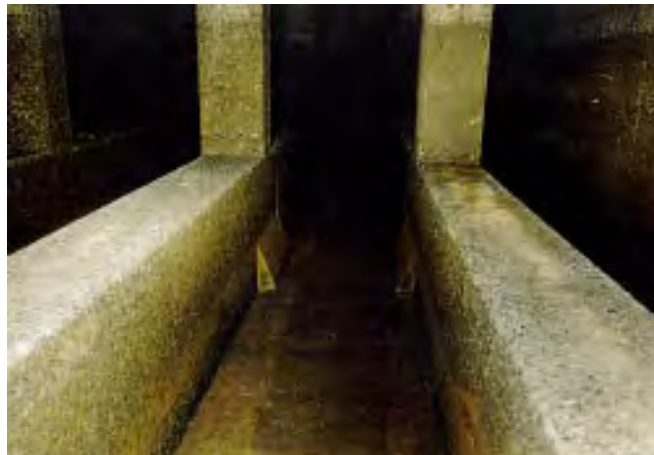
Figure 5. Fuel Basin floor, divider walls (curbs), and columns.
