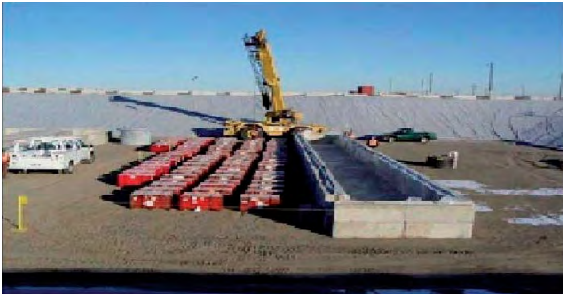
Figure 8: LLW facility at the Hanford site.
