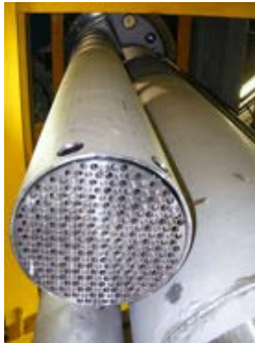
Figure 26: View of the ICE HX installed into the test section.
