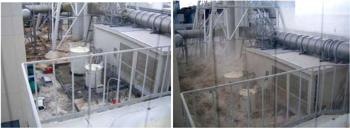
Figure 22 - Water waves ingress at the base of the ventilation stack system
