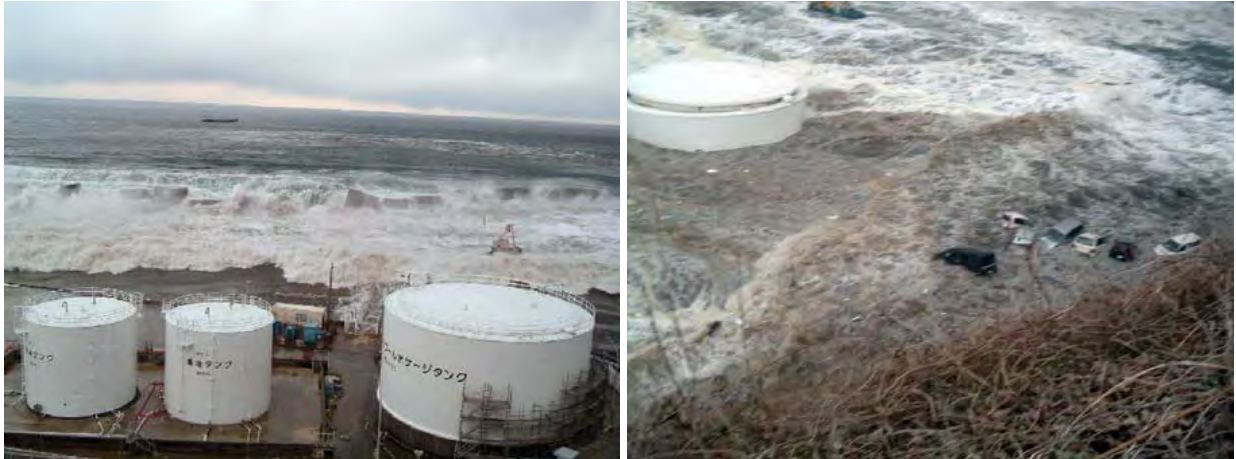
Figure 21 - Tsunami waves impinging on the 6 m protective wall of the nuclear plant
