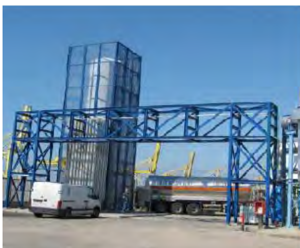
Figure 5 Refill of the oxygen storage tank
