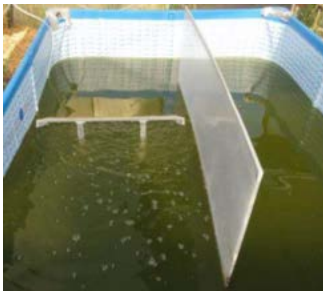
Figura 13. Air lift a piano inclinato
