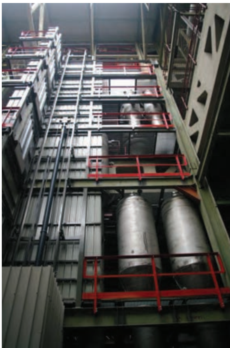
Figure 7 – SPES 3 steel structure
