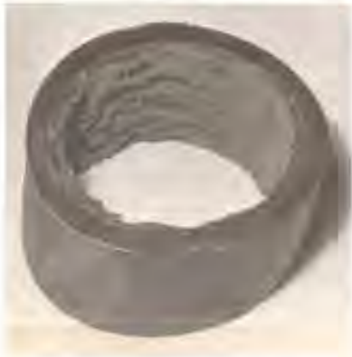
Slag in pipeline
