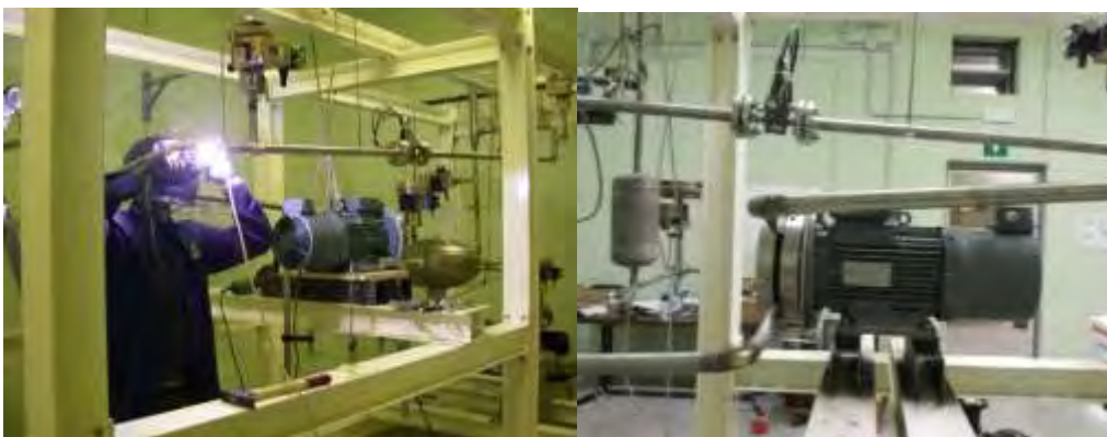
Figure 4 - installation of the pump and final configuration
