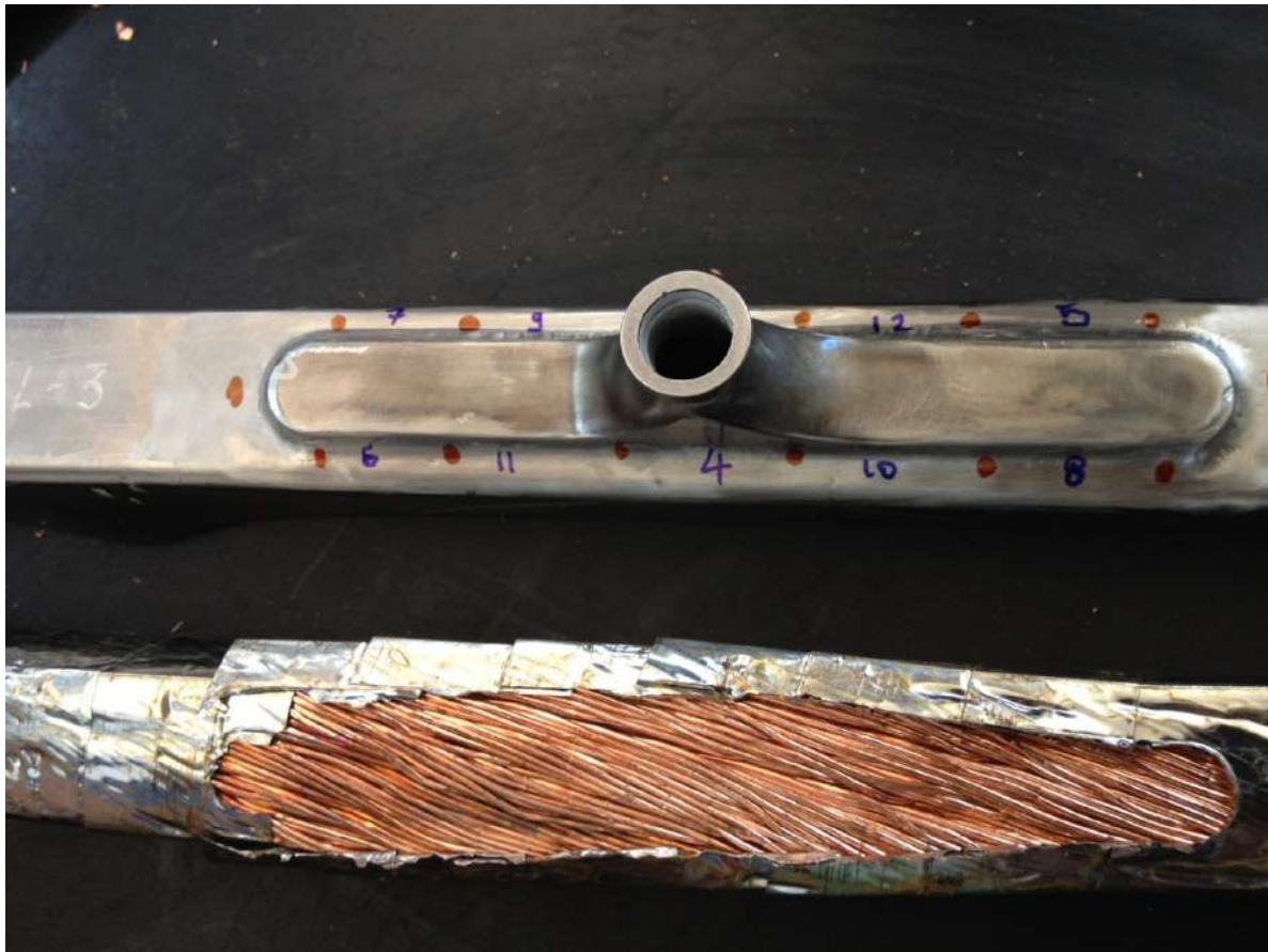
Fig. 5 Appearance of cable after extraction.
