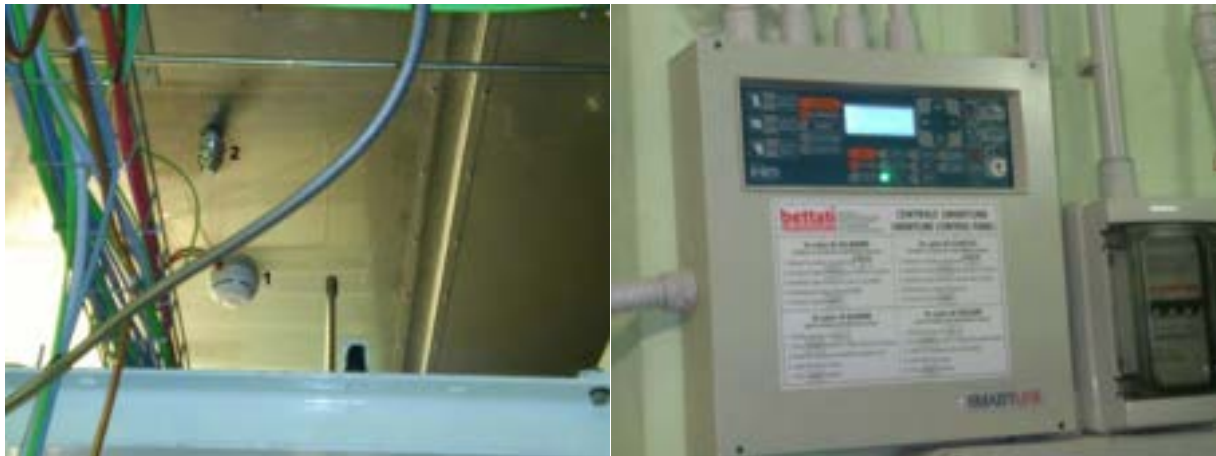
Figure 11: left: inner view of part of the top of the containment box (1: one of the four smoke detectors; 2: one of the two Argon injectors); right: dedicated control panel of the fire extinguishing system
