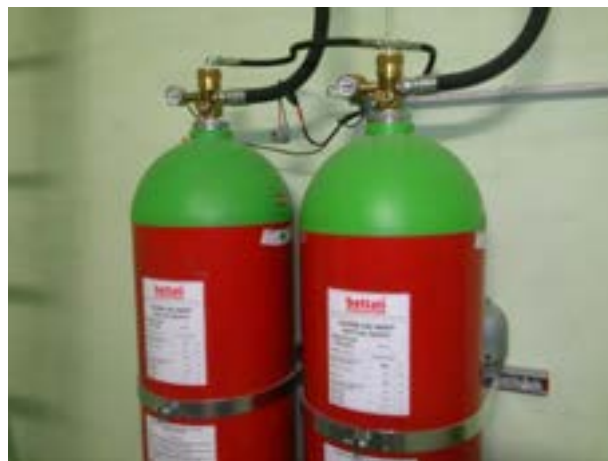
Figure 12: Dedicated high pressure Argon cylinders for the fast injection in the safety box
