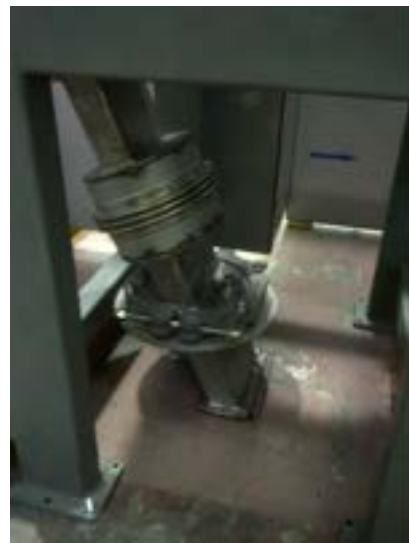
Fig. 23 The bellow on the outlet channel
