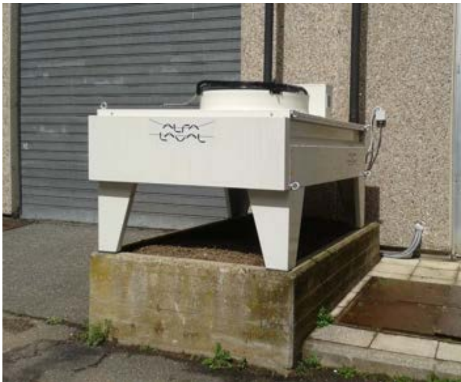
Figura 10. Dry Cooler Alfa Laval
